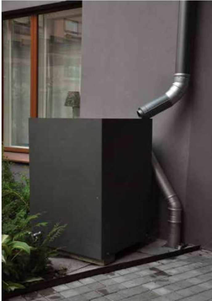
Figure 87: Examples of tanks used for rainwater harvesting.
