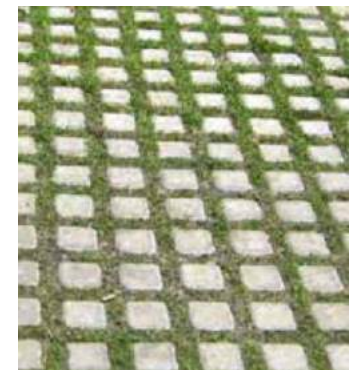
Figure 91: Permeable concrete paving.
