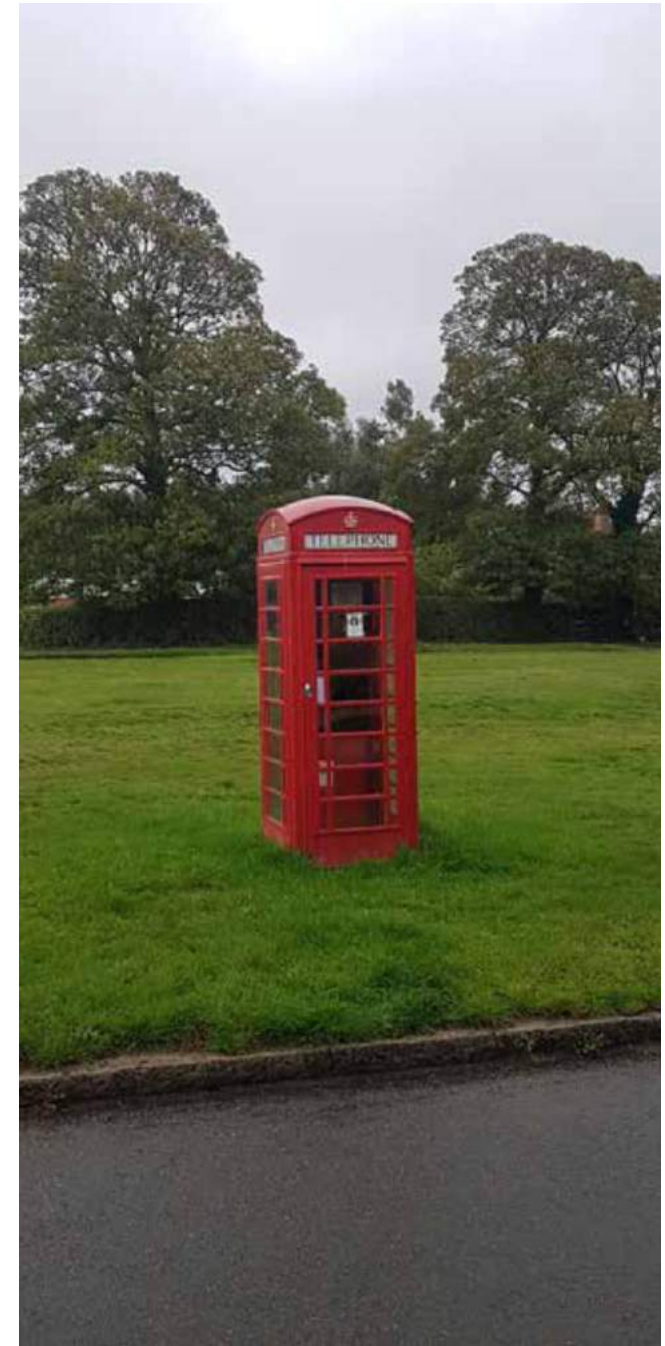
Figure 13: Grade II listed K6 telephone kiosk located on the Green.
