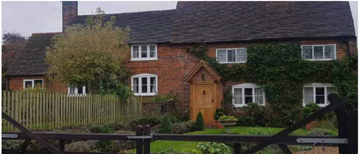
Figure 70: Traditional house with upper floor horizontal sliding multi-pane sash windows and ground floor casement windows with cambered heads.
