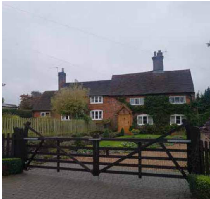
Figure 11: Red brick building with clay plaintile roof.
