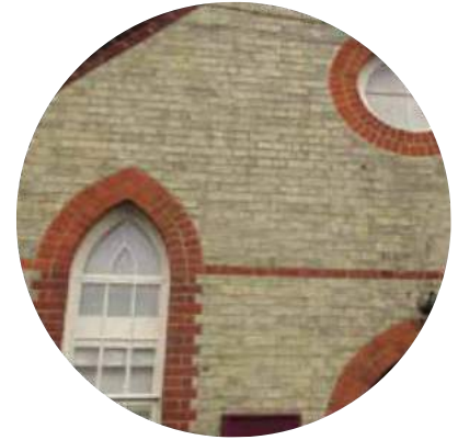
Red brick trim and yellow brick infilling
