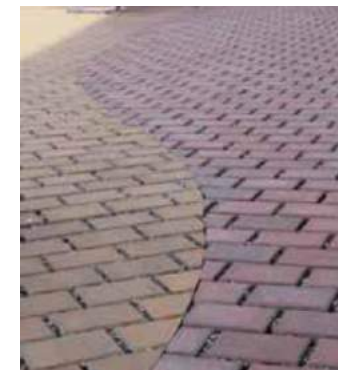
Figure 90: Permeable brick paving.
