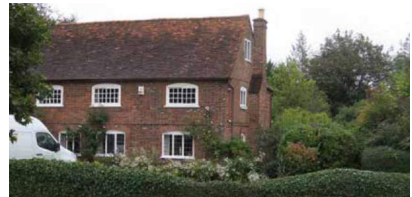
Green End Farmhouse – red brick façade with upper floor horizontal sliding sash windows and ground floor multi-paned casement windows with cambered heads.
