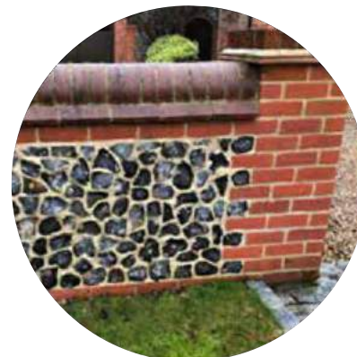
Knapped flint and red brick boundary wall
