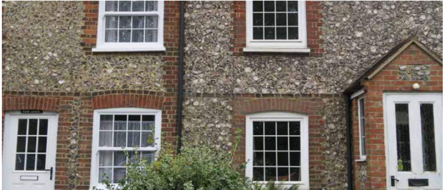
Figure 69: Façades with a consistent arrangement of multi-pane windows with attractive brick ornamentation and articulations.
