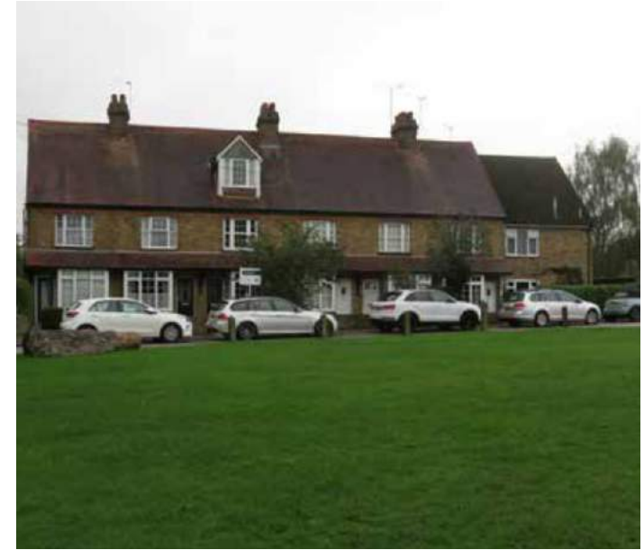
Figure 16: Terraced cottages on the Green with little building setback.
