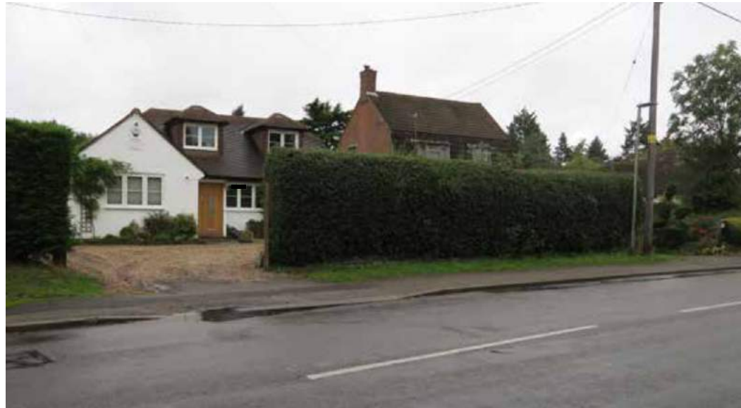
Figure 52: Gravel front yard parking with landscaped property boundaries preventing a car-dominated character.
