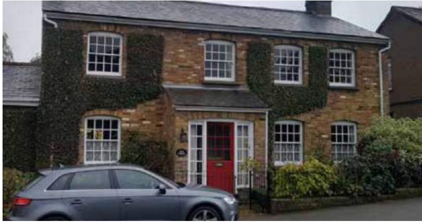
Yellow stock brick house with a symmetrical elevation emphasised by an even distribution of sash windows and consistent treatment of window details.
