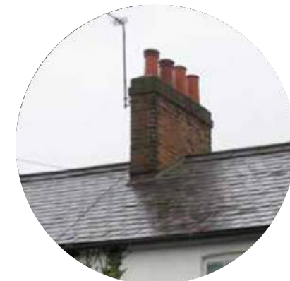
Red brick chimney
