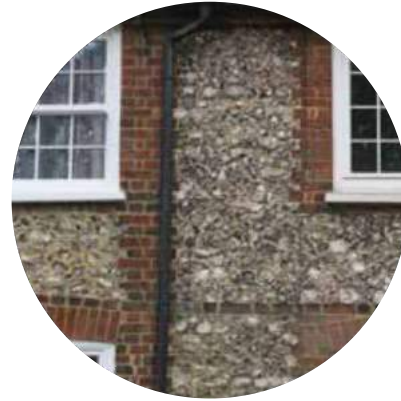
Red brick trim and knapped flint infilling
