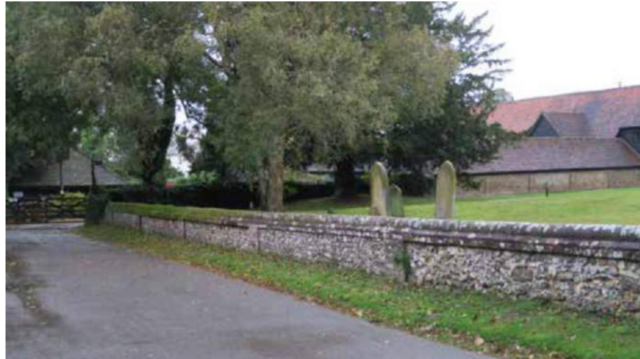
Figure 72: Church yard wall built with local flint.
