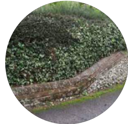
Low masonry wall with landscaped hedge
