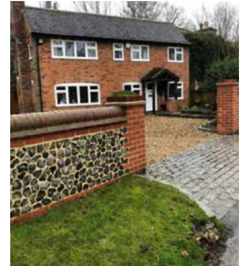
Figure 73: New wall using a mix of traditional local materials © Sarratt Parish Council.
